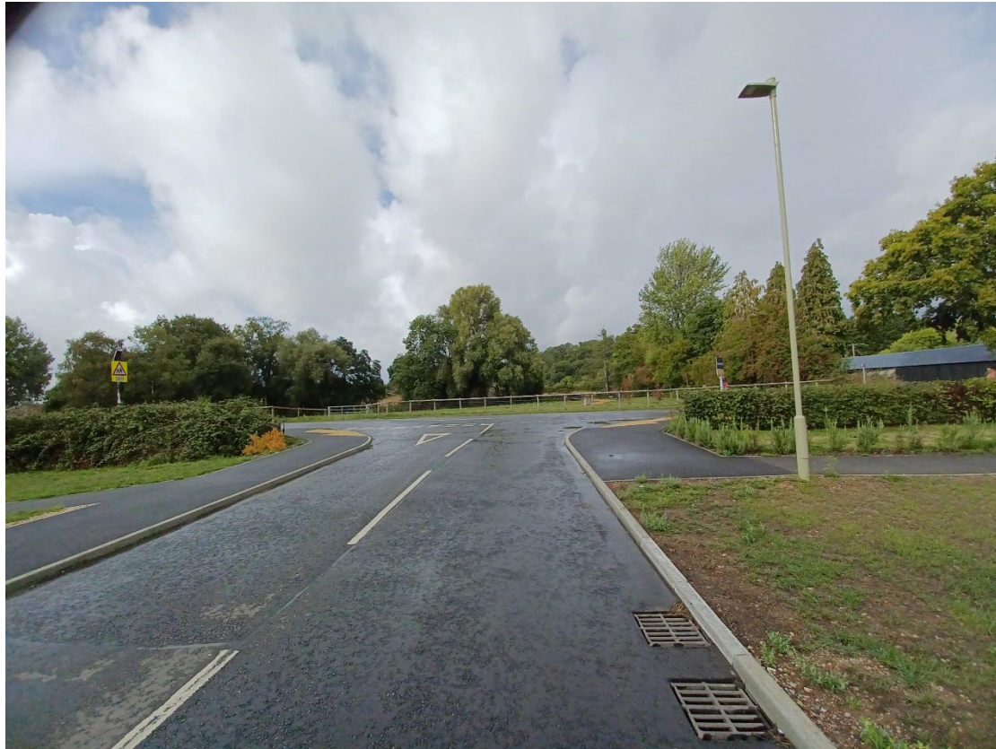
Looking towards Whitsbury Road and point of new roundabout and site access from Augustus Park
