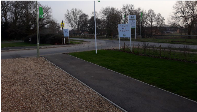
Roundabout and accommodation works
